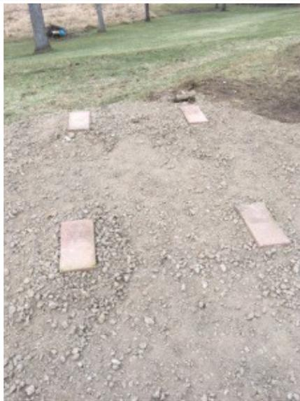
*Use 4 solid concrete blocks on firm level ground*
